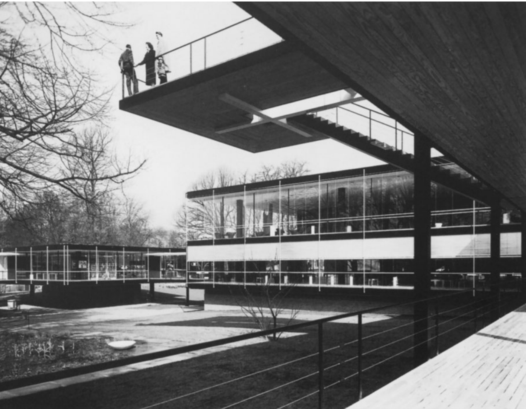
The West German pavilion at the Brussels World Exhibition 1958 by Egon Eiermann
